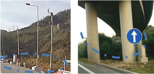
**Fig. 6** Unprotected lighting and road sign poles and bridge pillar
