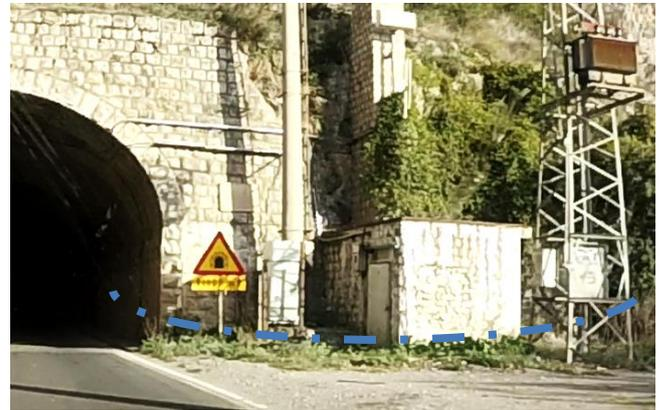
Fig. 2 Unprotected obstacles at a tunnel portal
