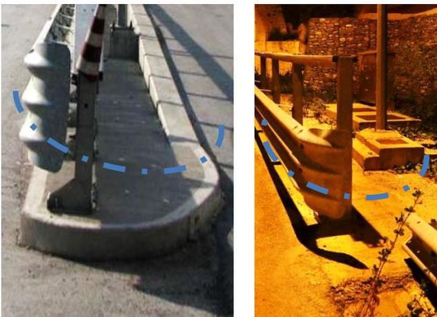
**Fig. 8** Inappropriate guardrails finishing/ Interrupted guardrails
