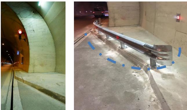
**Fig. 9** Installation of guardrail in front of perpendicular wall of lay-by in Krrabe tunnel in Albania (before and after situation)[10]
