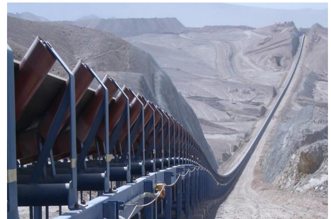
Fig.1. View of a long overland belt conveyor
