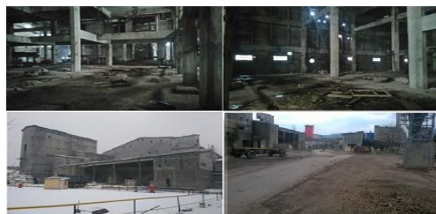
Fig. 6 The current state of the building
