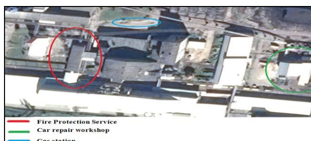
Fig.5 Display of the outbuildings next to the Central Warehouse
